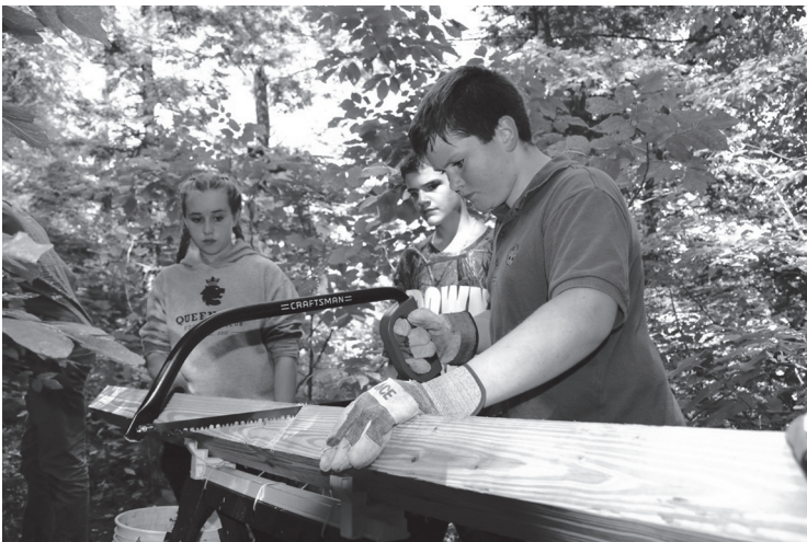
Building a new foot bridge at Round Pond Natural Area
