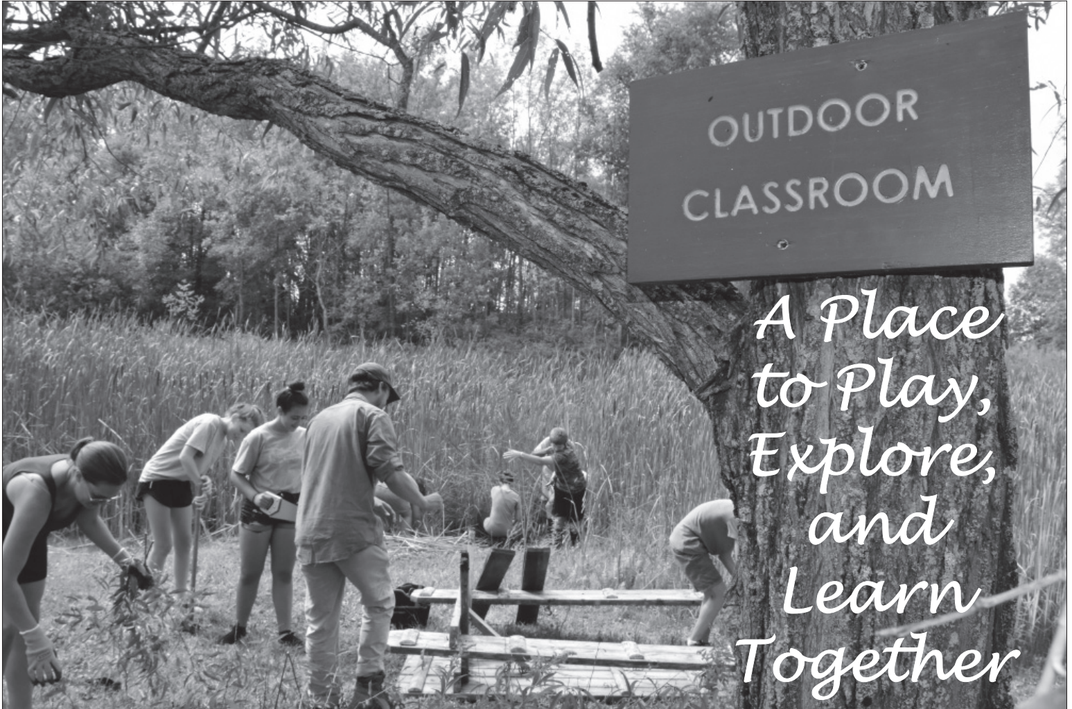
Middle school students repair a picnic table and clear cattails at the pond behind the school. Photo credit: Rob Swanson
