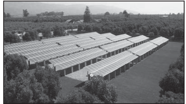
Solar photo-voltaic tracking system, photo courtesy of: http://www.gosolarcalifornia.org/about/images/csi_solar_array.jpg
